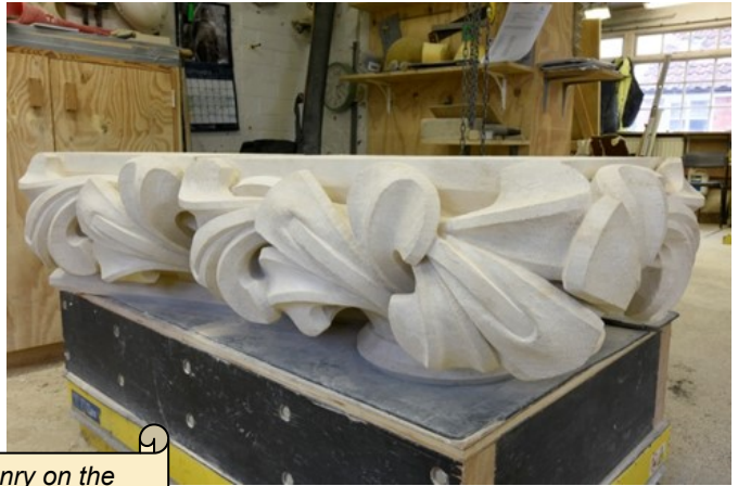
Decayed masonry on the North Choir Aisle, and its replacement with stiff leaf carving ready to be fixed
