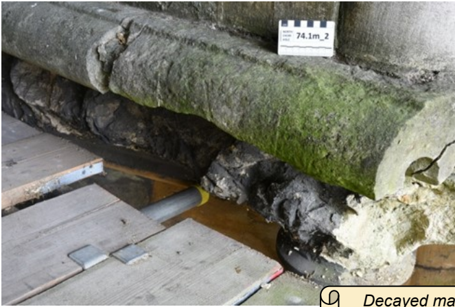
Decayed masonry on the North Choir Aisle, and its replacement with stiff leaf carving ready to be fixed
