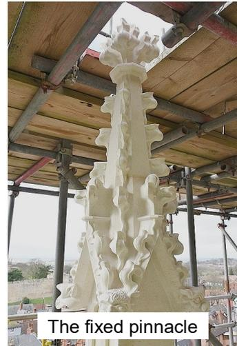
The masonry towards the bottom of the Turret is less decayed than the stones higher up. The majority of the work in this last year of the project is consolidating and preserving the original stonemasonry, including conservation cleaning of the existing carvings.
